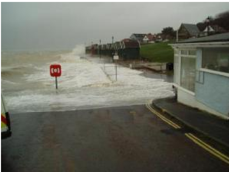
This image shows flooding at Gurnard on the Isle of Wight, UK. (Credit: Centre for Coastal Processes, Engineering and Management)
